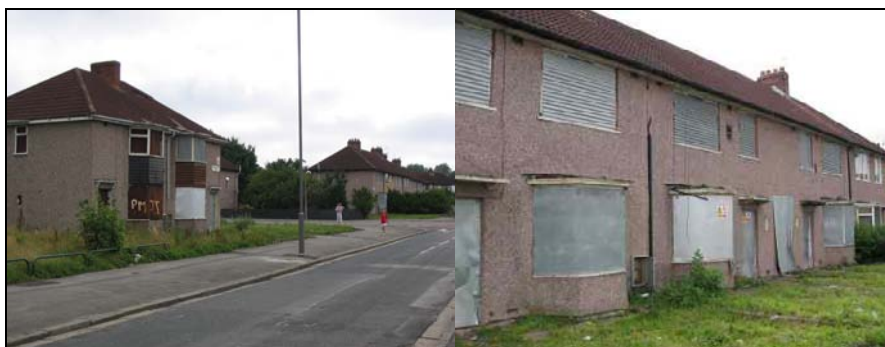
Figure 5.1 Row houses under demolition next to inhabited houses in a deprived ward (Alt Valley - North Liverpool)
