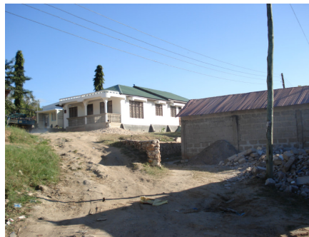
Figure 5.15: Complete house in Kimara
