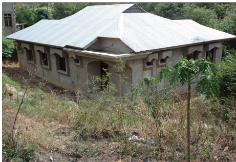
Figure 5.14: House under construction in Kimara
