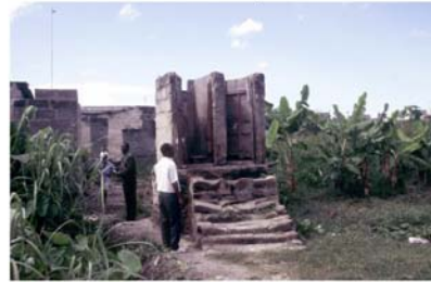
Raised latrine in flood plain
