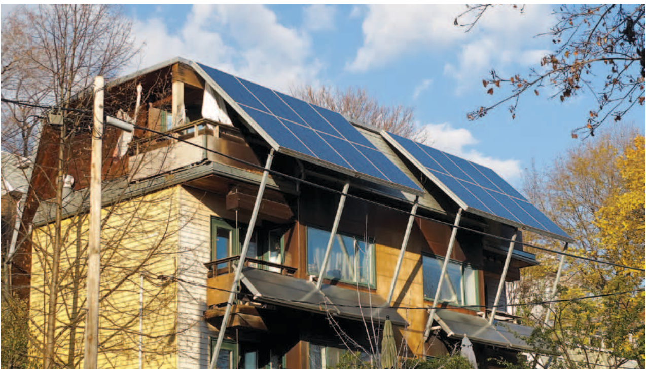
● New networked technologies involve decentralising energy production, consumption and savings management
